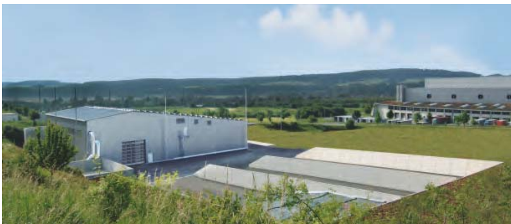
The new biogas system shortly before start-up. 4,500 tonnes of various substrates are transformed here into more than 500,000 cubic metres of biogas annually.
