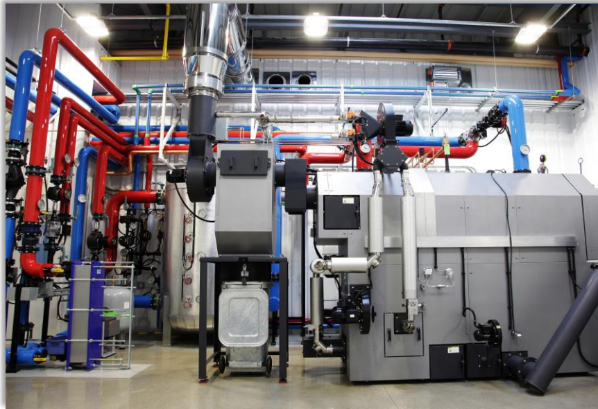
Viessmann Canada, Waterloo, ON Biomass boiler plant with Vitoflex 300-UF (output: 1330 MBH)
