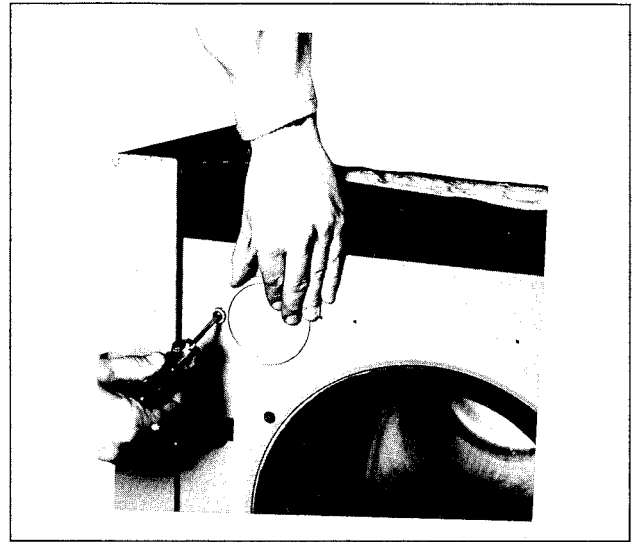
Securing the capillary sensors by re-installing the cover plate over the 5-point stainless steel well.
