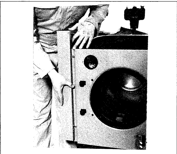
Align panel slots with hex. bolt heads. Push side panel towards boiler - press - panel towards boiler rear and down to hook in place.
