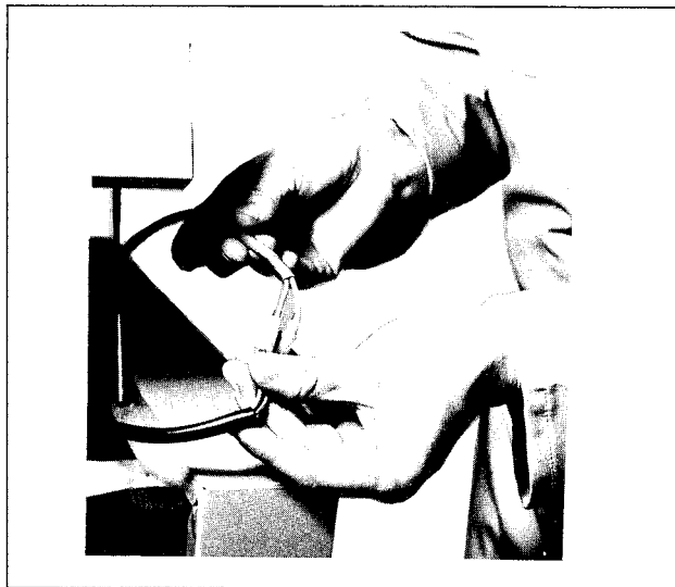
Making the operating control connection (room thermostat, indoor/outdoor control, etc.).
