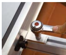
Site and secure the first collector
