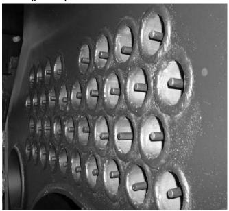
Insert the displacement rods into the heat exchanger tubes with the thick end first. Push until they are flush with the edge of the tube. Tolerance  $\pm 1/4$  (5 mm).
