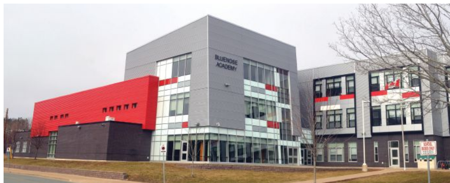
When the Grade P-9 school in Lunenburg, N.S., was built seven years ago it was the greenest building in Atlantic Canada and achieved LEED Gold certification.
