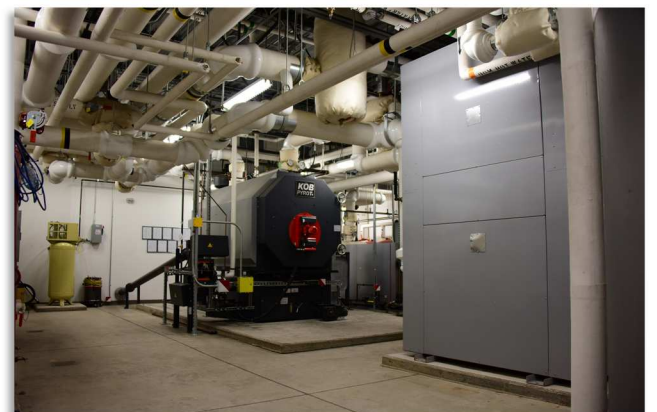
Viessmann Pyrot KRT-540 wood pellet boiler (1843 MBH)
