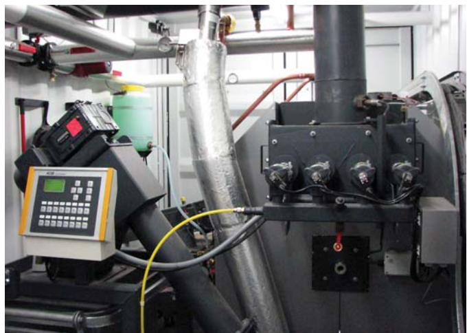
The fully-automated boiler system utilizes modern combustion technology, advanced safety systems and digital controls to deliver clean, reliable and efficient biomass heating
