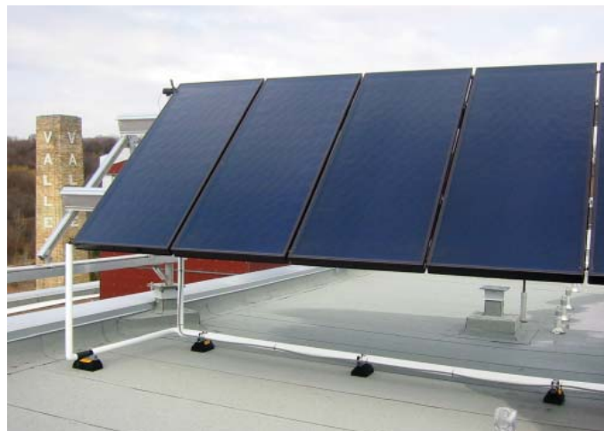
Vitosol 200-F collectors offer supplementary heating for up to 50% of the CGC's DHW supply
