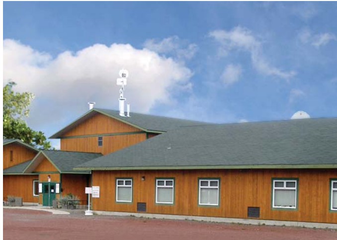
The new biomass heating system displaces approximately 130 tonnes of CO 2 annually
