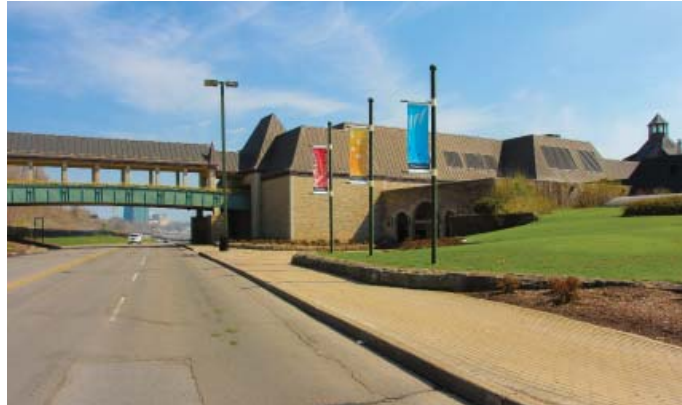
The ice and snow melt system keeps the pedestrian walkway and main entrance clear
